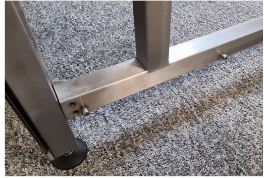
2 - Fit cap-head screws at base level
